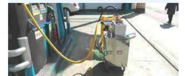
Pressure Reduction, Leakage Inspection
