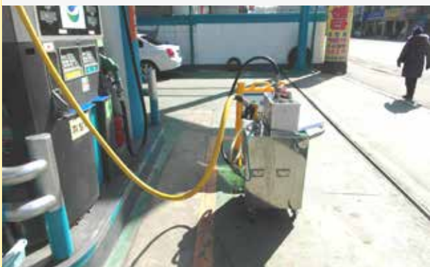
Pressure Reduction, Leakage Inspection
